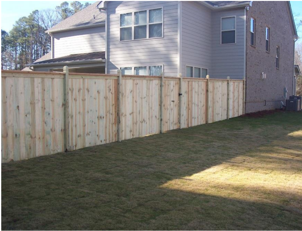
Cap Top Privacy Fence
